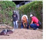
Installation of drip lateral
