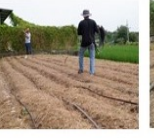
Installation of drip tape
