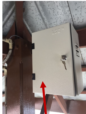
Metal Box installed at UTM/FABU bus stop
