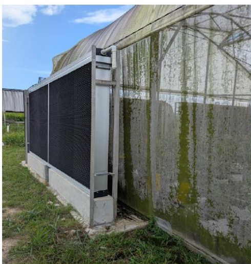
Figure 1a – Inspecting the waterwall installation.
