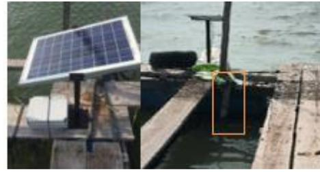
**Figure5. Complete solar-powered panel box installed with cylinder pipe and soaked in the seawater.**
